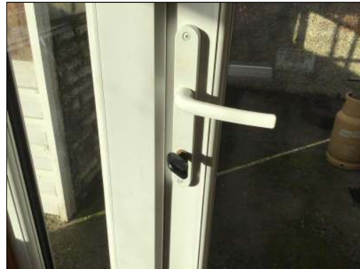
Photo - 86 Lock not secure
