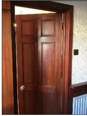
Photo - 48 Typical door and frame
