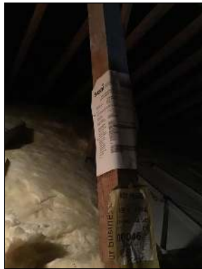
Photo - 25 Insulation SEAI Certificate.
