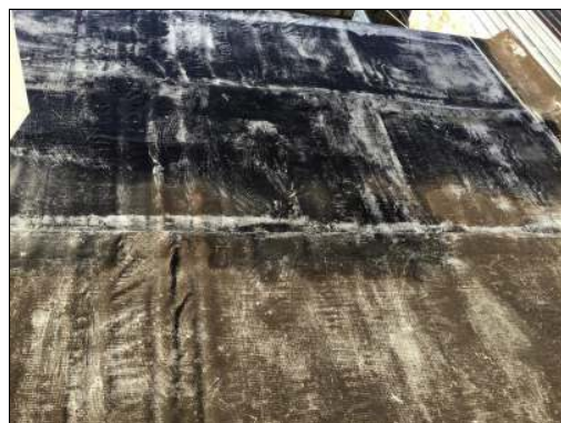
Photo - 3 Flat roof over extension
