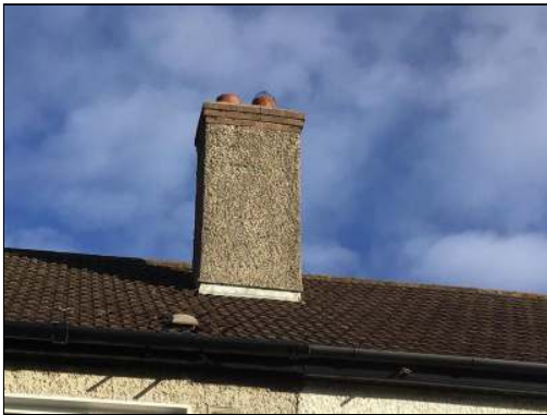
Photo - 1 Chimney to rear.
