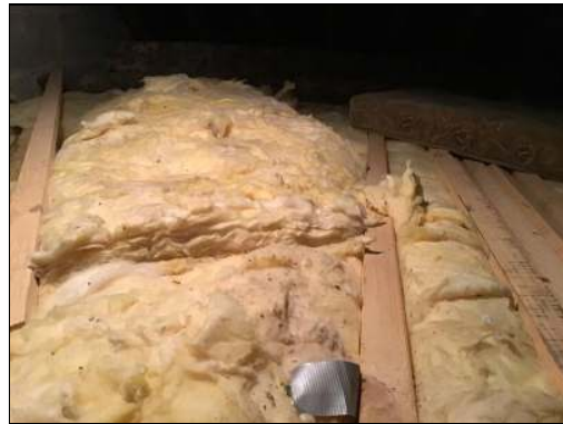
Photo - 24 Rockwool insulation
