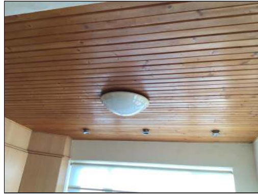
Photo - 30 Panelling on ceiling in kitchen
