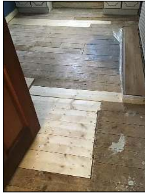
Photo - 40 T&G flooring in bedrooms
