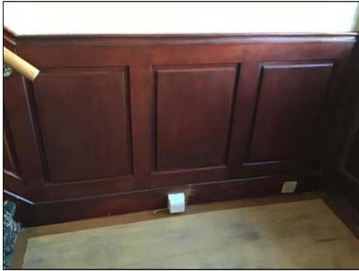
Photo - 50 Wainscoting in hall and along stairs
