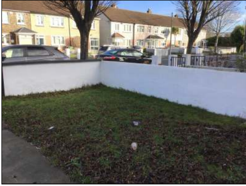
Photo - 22 Front boundary wall
