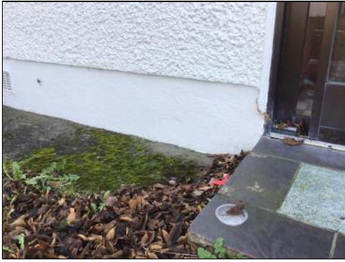
Photo - 54 Plinth and front step
