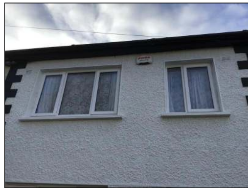
Photo - 13 Typical window
