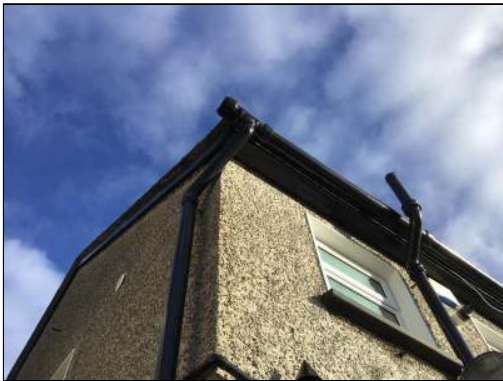
Photo - 6 Rain water pipes and gutters
