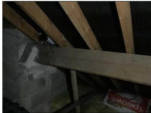
Photo - 26 Additional collar ties to be fitted
