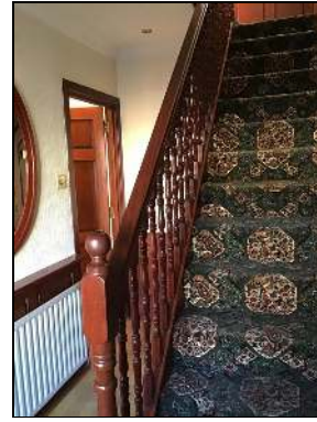
Photo - 49 Hardwood stair rail
