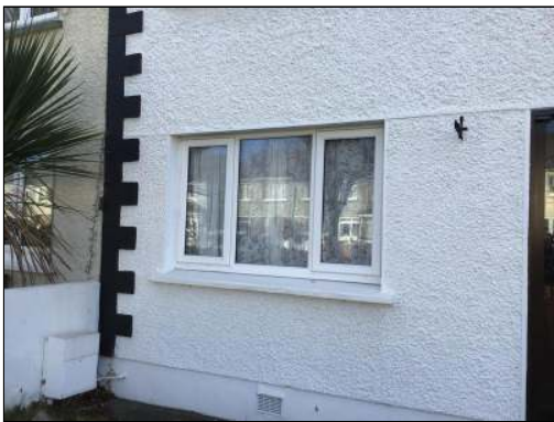
Photo - 12 Typical window
