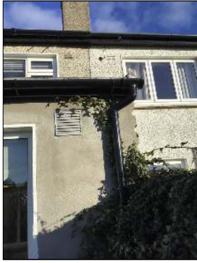
Photo - 4 Rain water pipes and gutters
