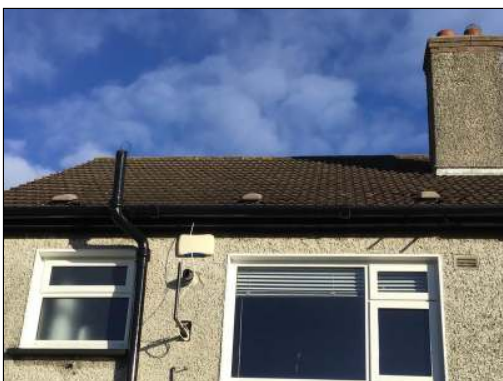
Photo - 2 Main roof
