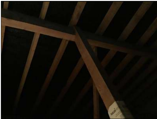
Photo - 23 Roof timbers in good condition
