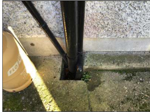
Photo - 71 Gully trap
