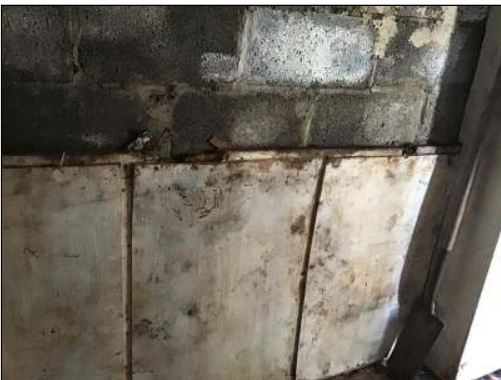
Photo - 83 Covered side passage to rear of shed
