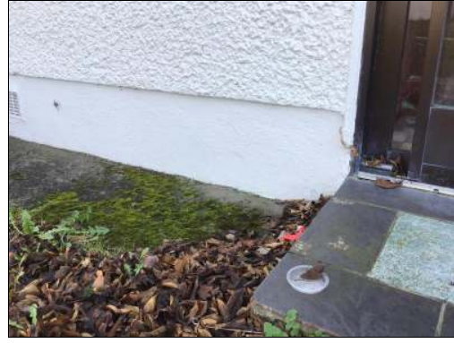
Photo - 11 Plinth and front step
