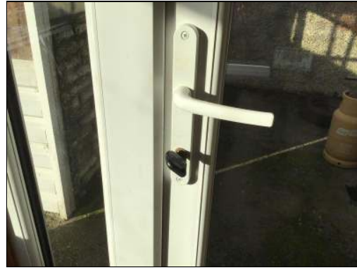
Photo - 17 Lock not secure
