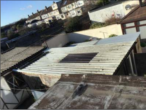
Photo - 79 Metal sheeting on workshop roof
